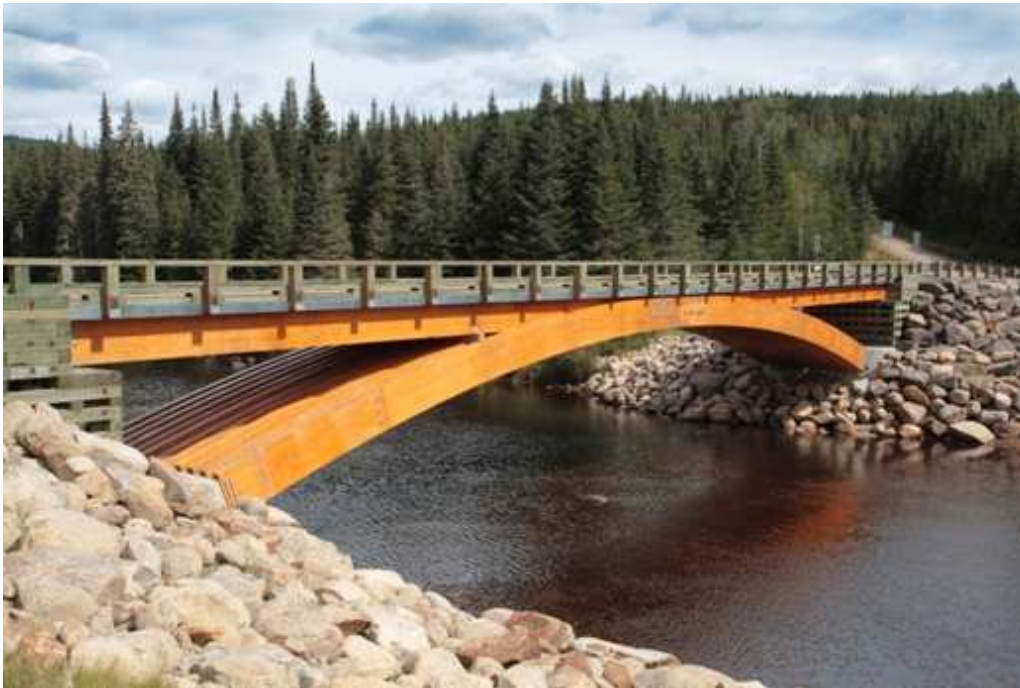
Figure 1 - Bridge located over the Montmorency river, in the Montmorency forest, Quebec, Canada. It has a span of 44 m, height of 33 m and width of 4.8 m [3].
